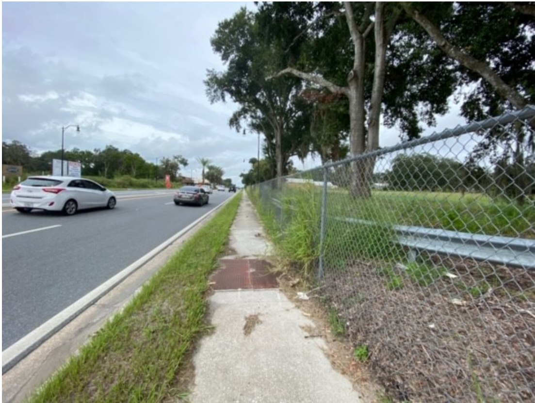
Looking west along East Dixie Avenue from sign posting.
