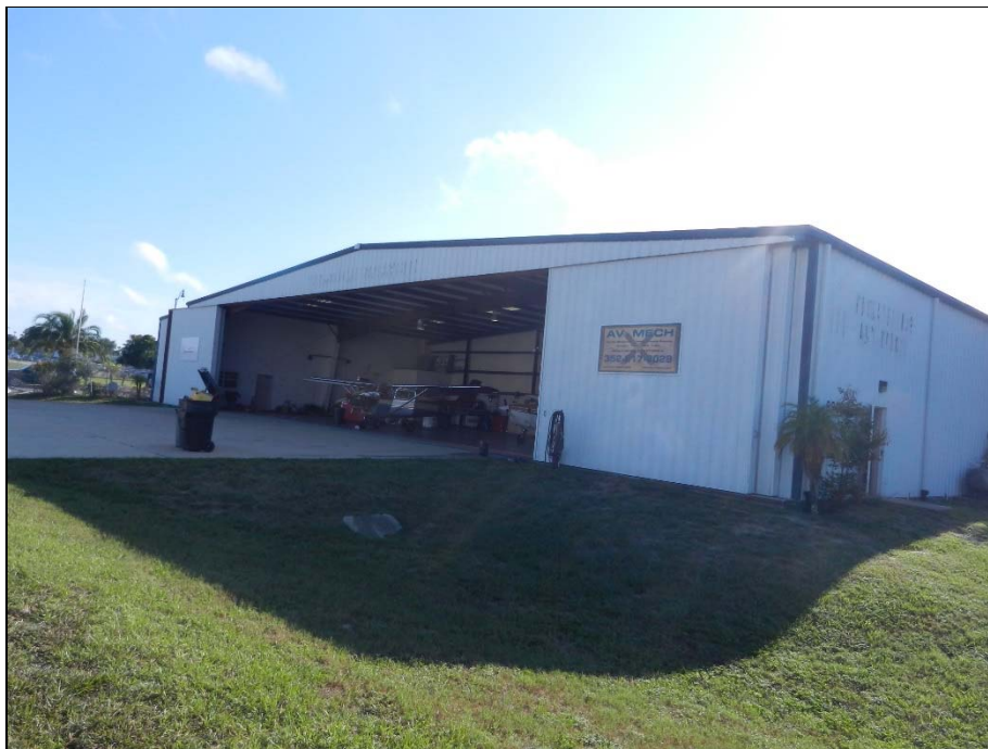
FRONT VIEW OF HANGAR
