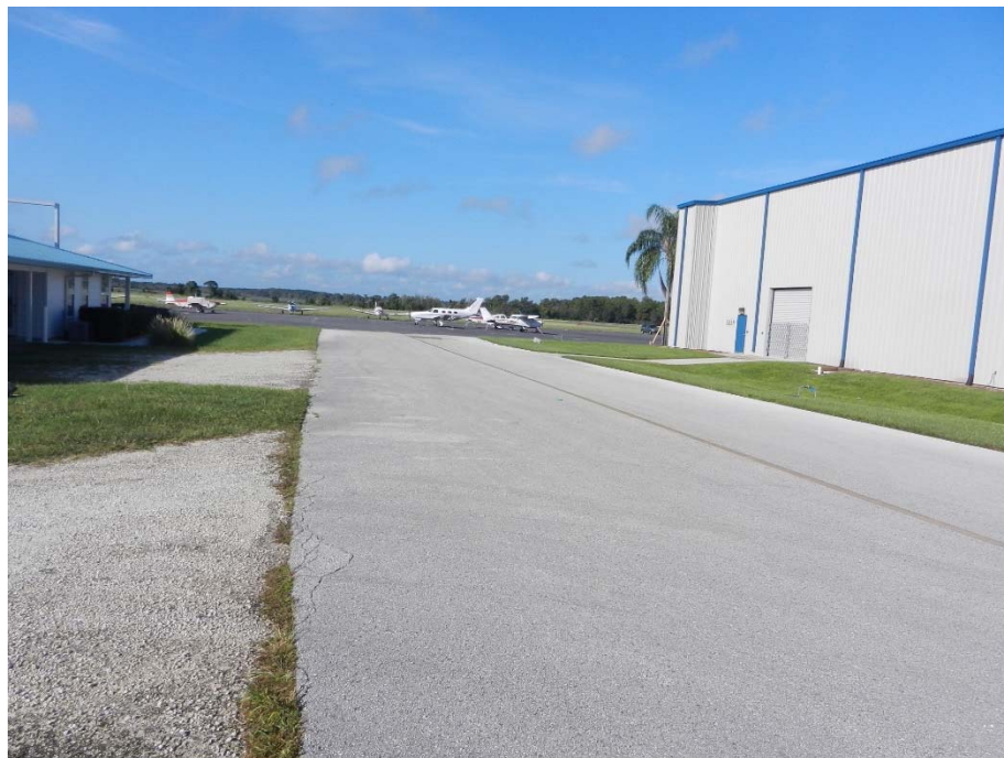
VIEW SOUTH ALONG TAXIWAY TO APRON (SUBJECT TO LEFT)
