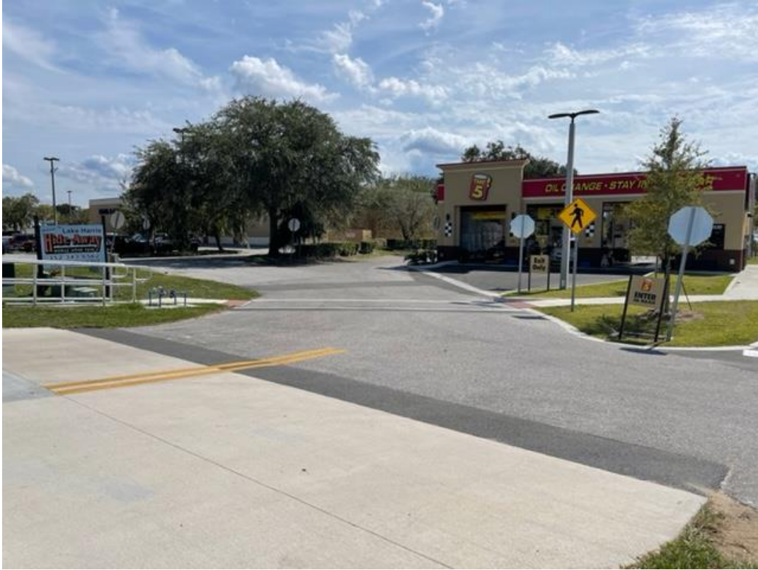
Looking south toward the property on Haven Ct from US Highway 441
