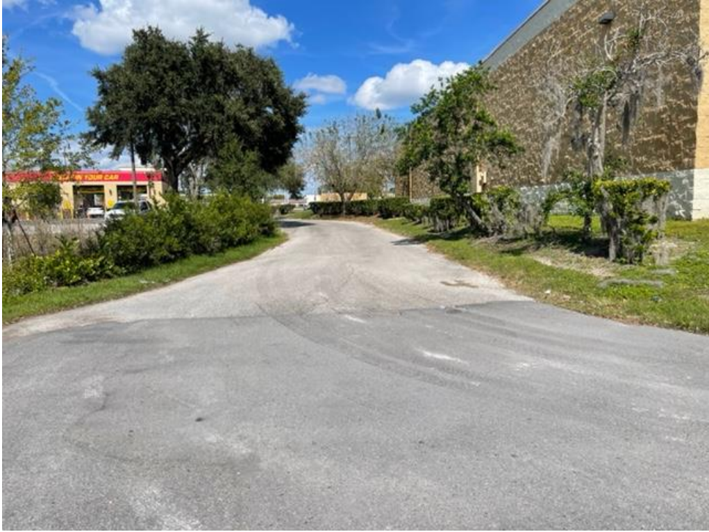
Looking north on Haven Ct
