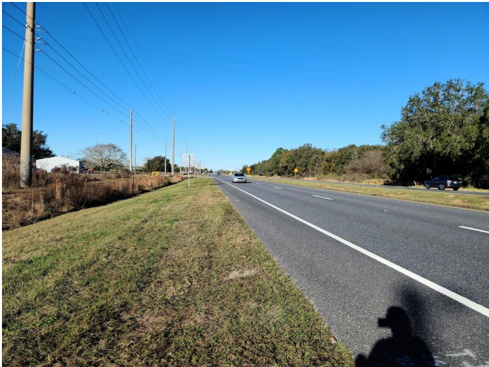
Looking west along SR-44
