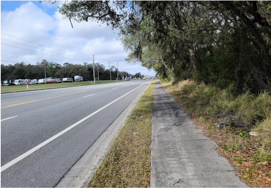
Looking west on W Main Street/FL 44.
