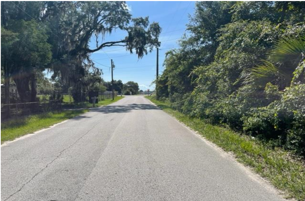
Looking south on East Treasure Island Ave
