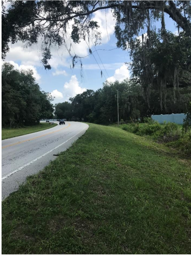
Looking north along County Road 470.
