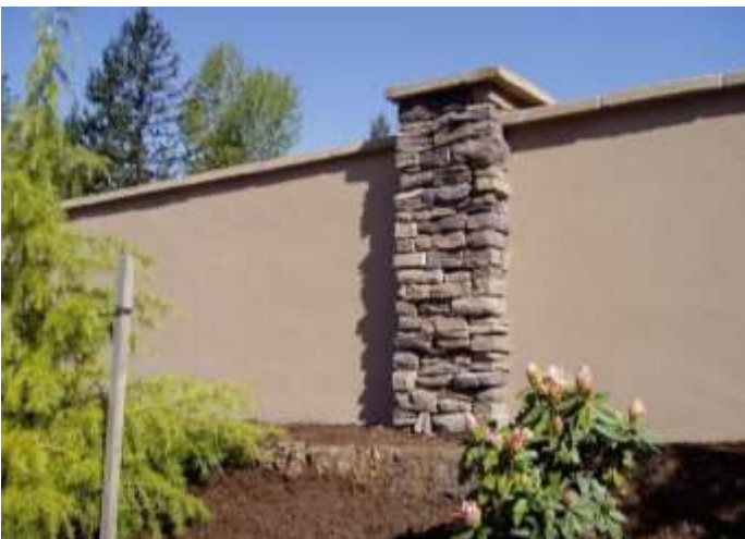
Figure 4– Opaque Wall with monument column features
