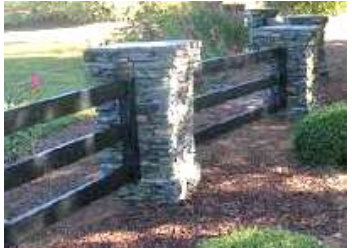
Figure 3 – Split rail fence with monument column features
