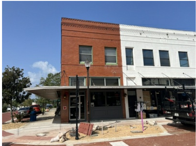
Typical view of subject
