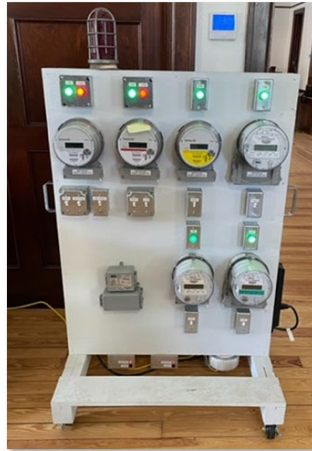
Figure 9. Example of Electric System Test Fixtures
