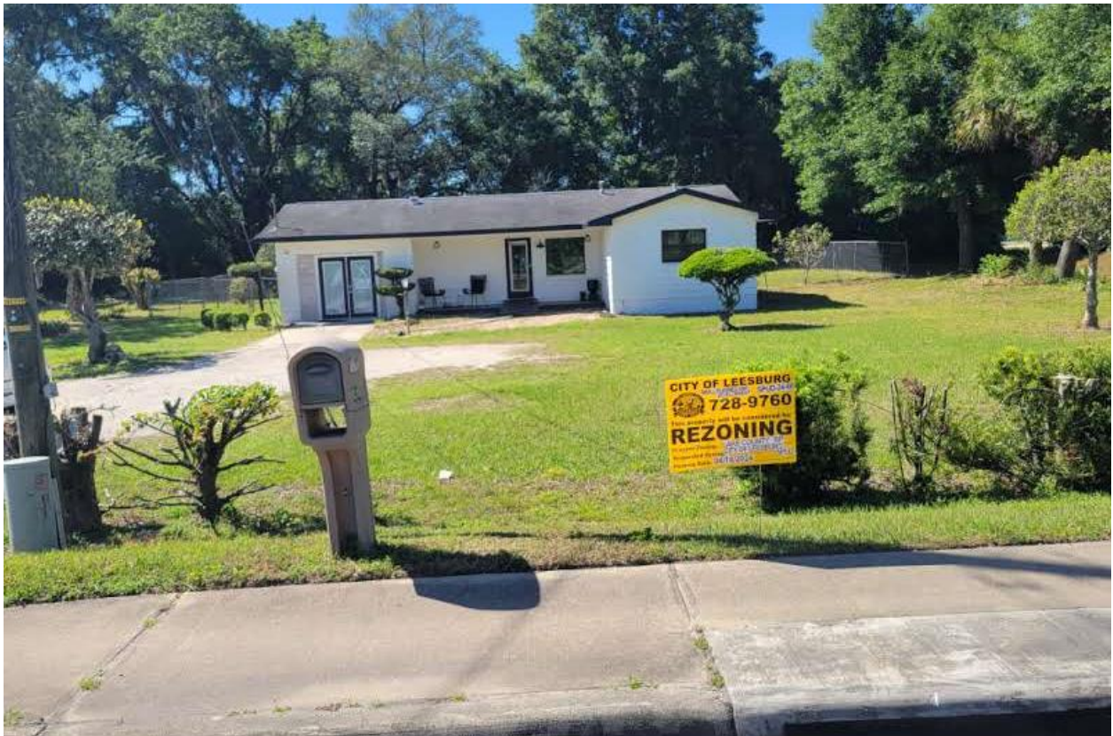
Looking South onto Subject Property from Griffin Road
