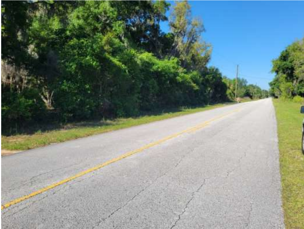
Looking west along Poe Street
