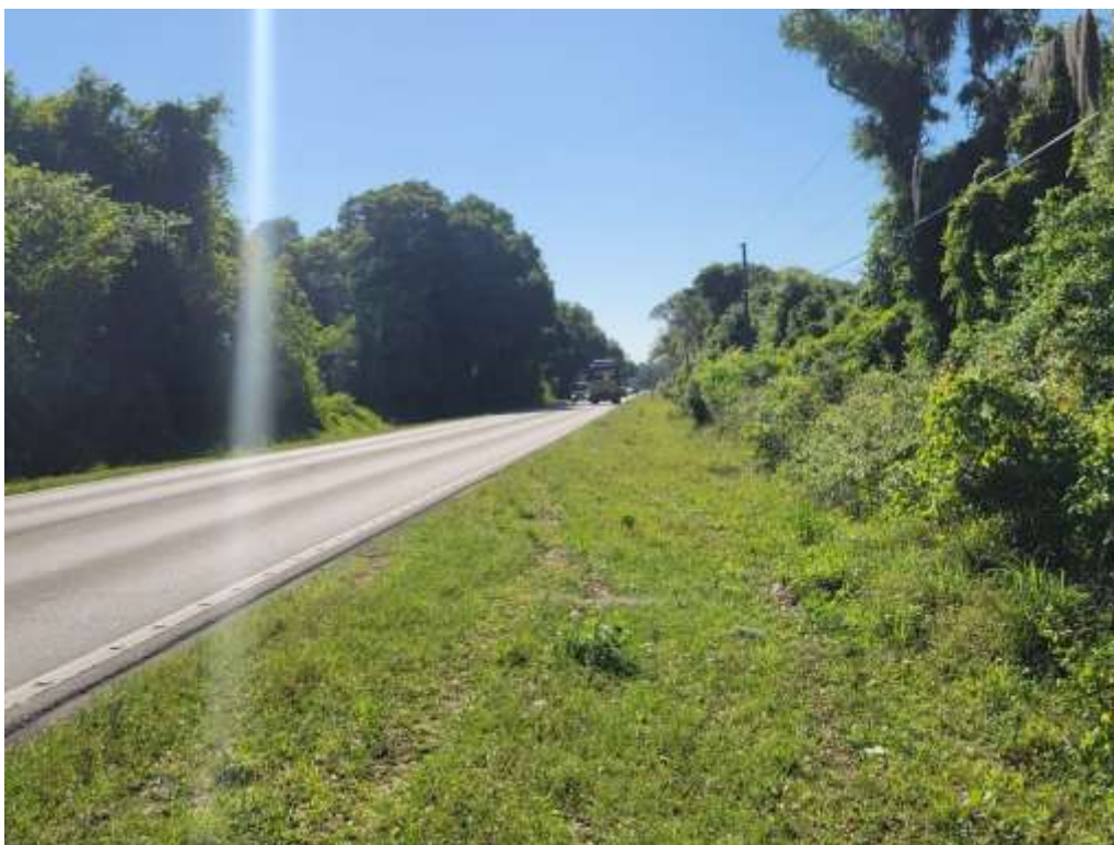
Looking southeast on County Road 473
