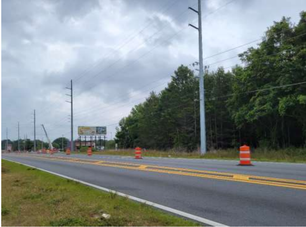
Looking east along County Road 48.
