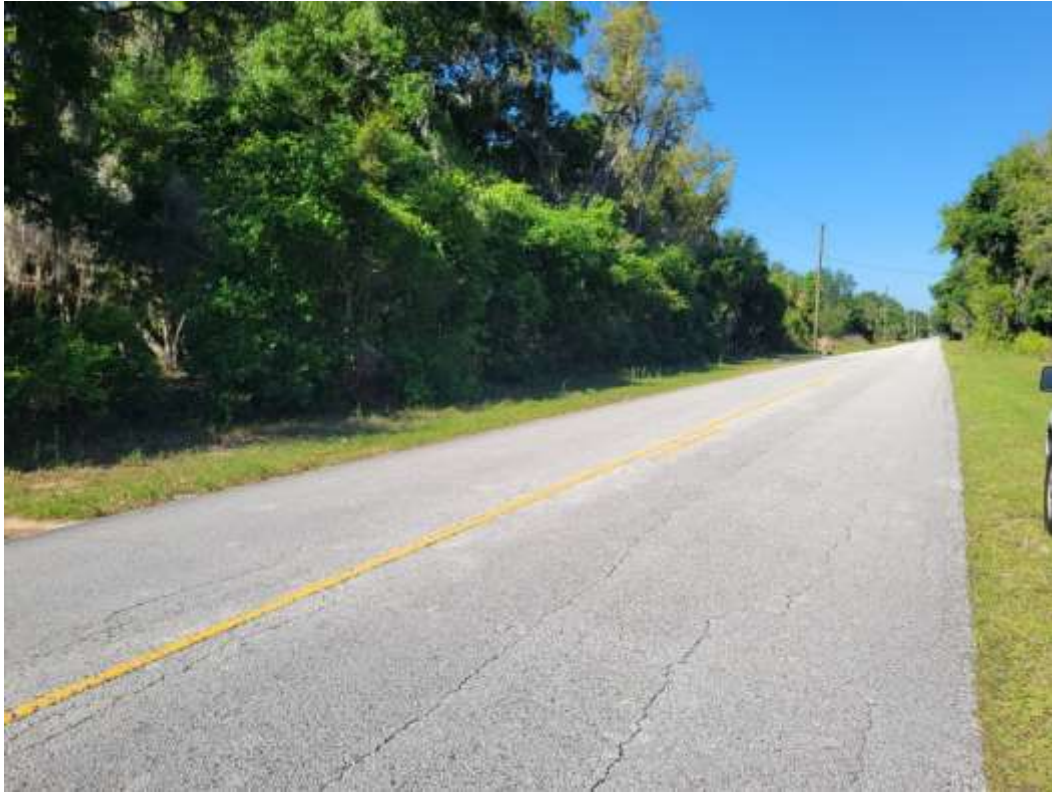
Looking west along Poe Street
