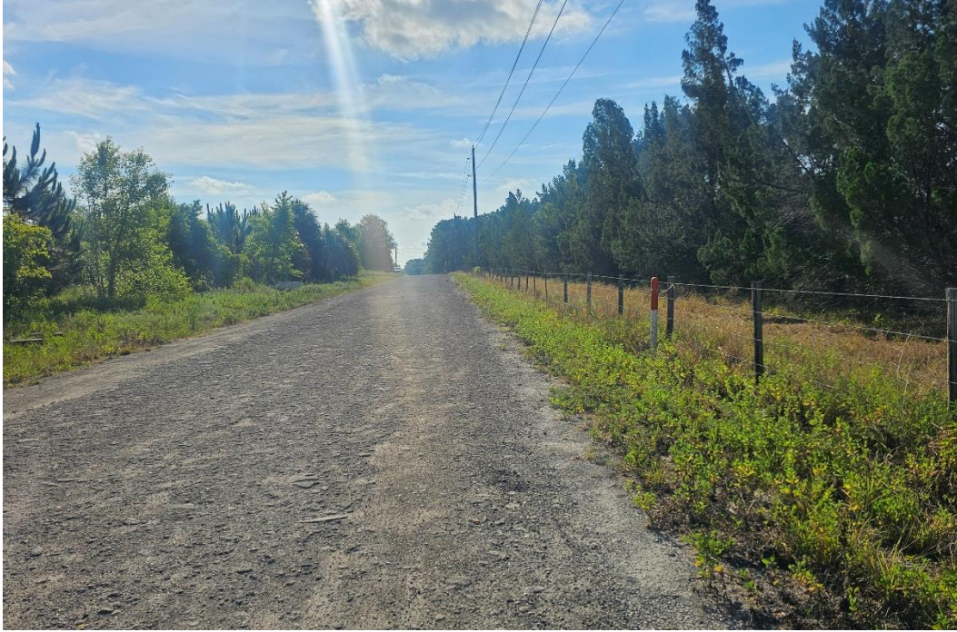
Looking east along Watson Road.
