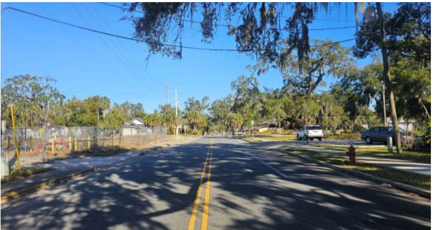
Looking North along Lee Street from Subject Property
