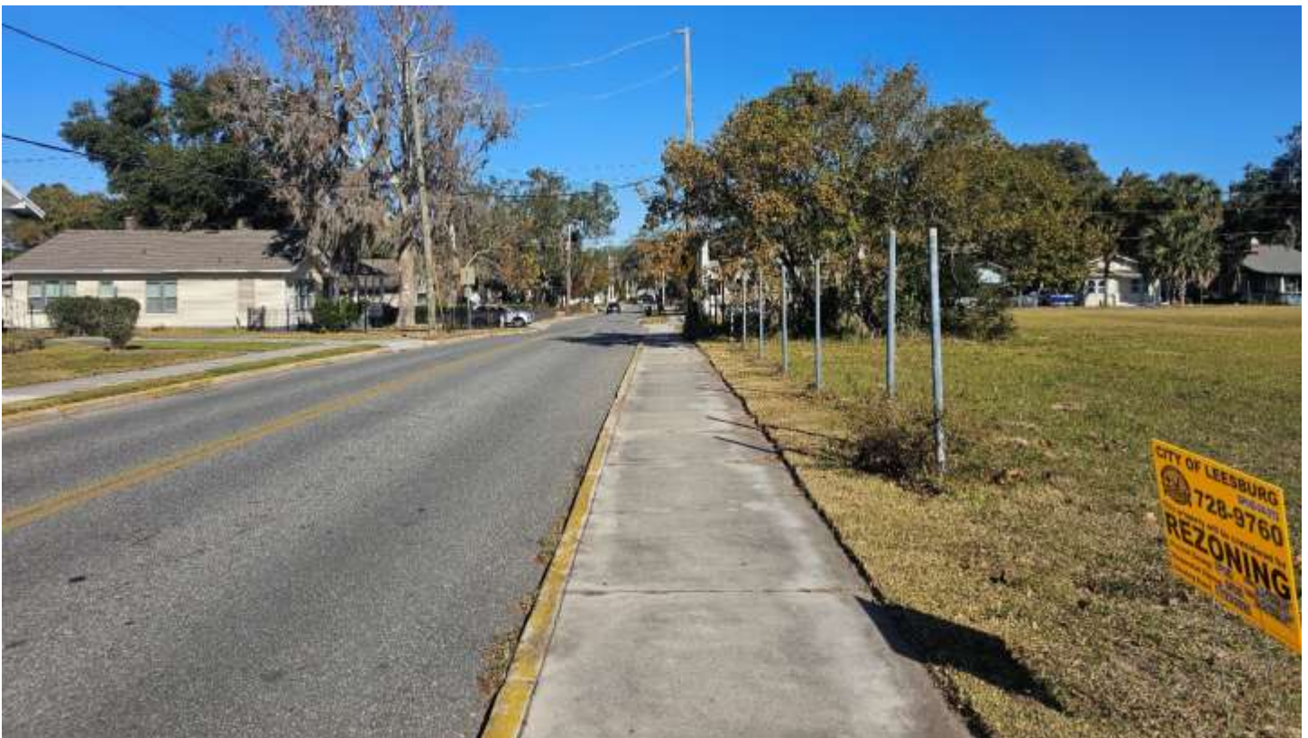
Looking North along Perkins Street from Subject Property
