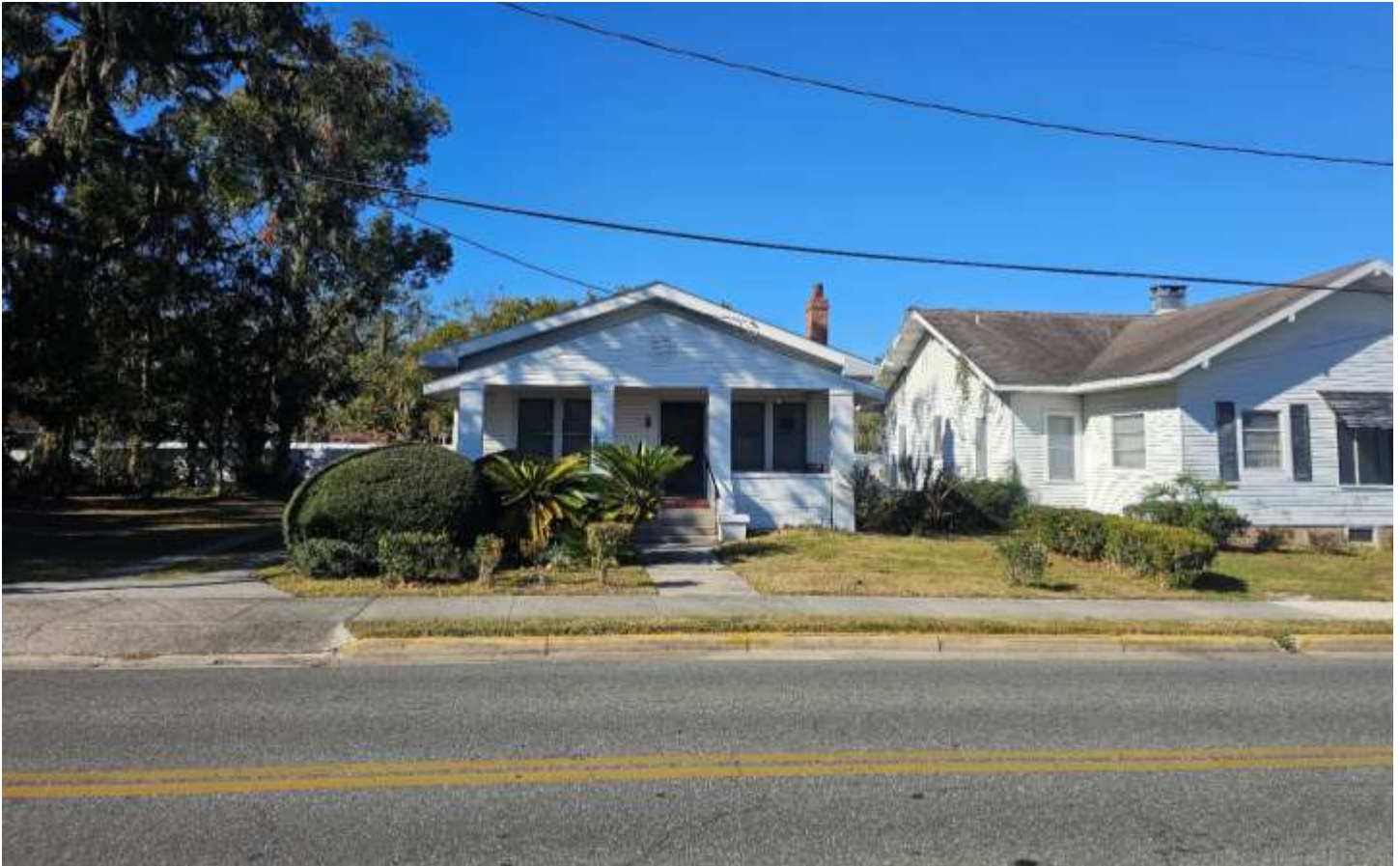
Looking West across Perkins Street from Subject Property
