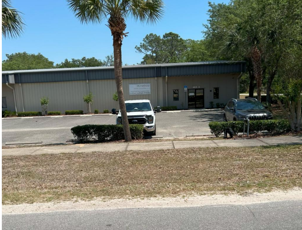
Looking east across Richey Road.
