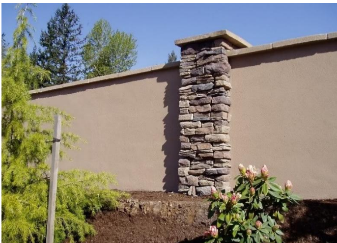
Figure 4– Opaque Wall with monument column features
