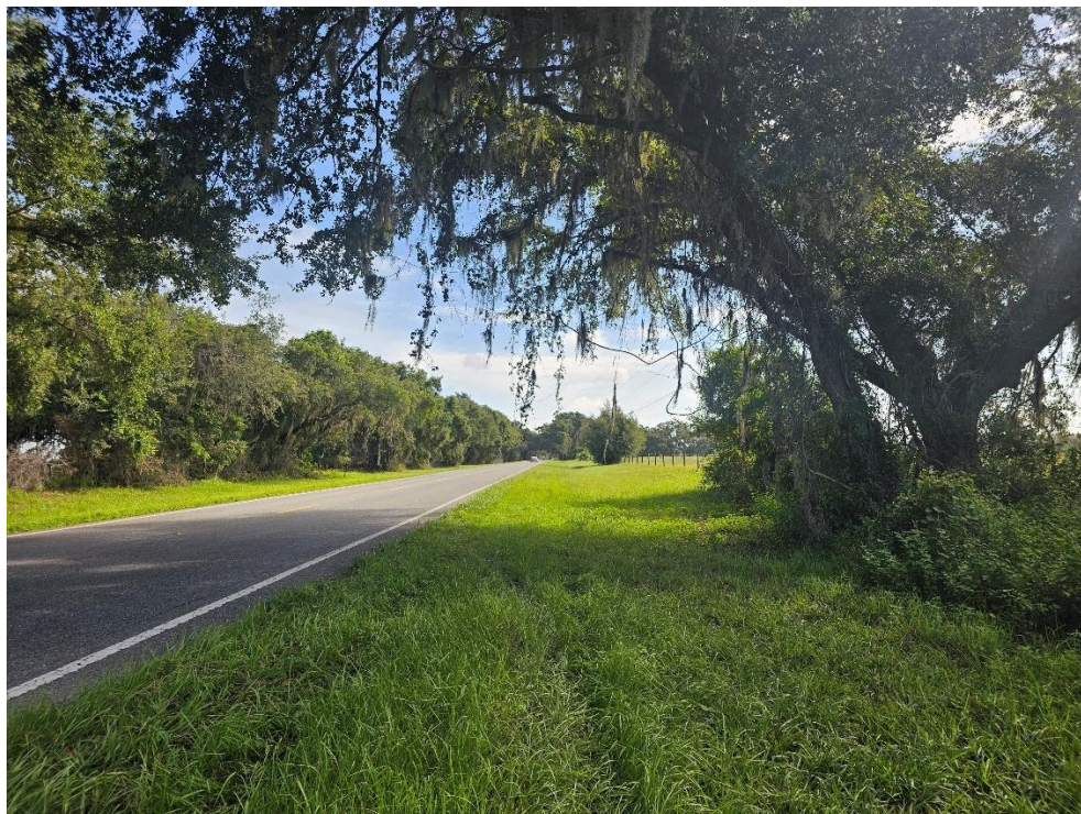
Looking North along County Road 48 from Subject Property.
