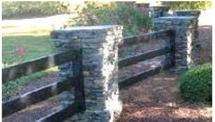
Figure 3B – Split rail fence with monument column features Example Source Courtesy of Fence & Deck Supply https://www.fenceanddecksupply.com/wp-content/uploads/2014/04/FDS-Mini-Product-Catalog-2014-EMAIL-.pdf
