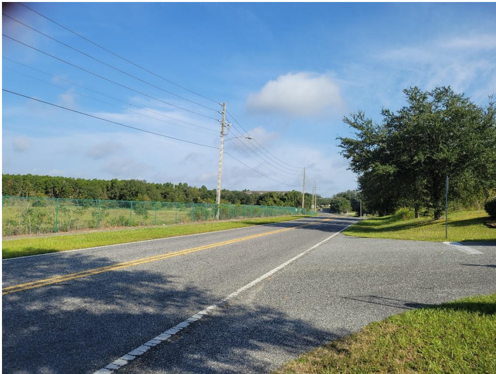
Picture taken from subject property looking north along Thomas Avenue.
