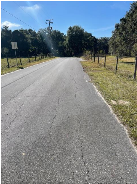
Picture taken from sign posting looking south along South Quarters Road right-of-way.
