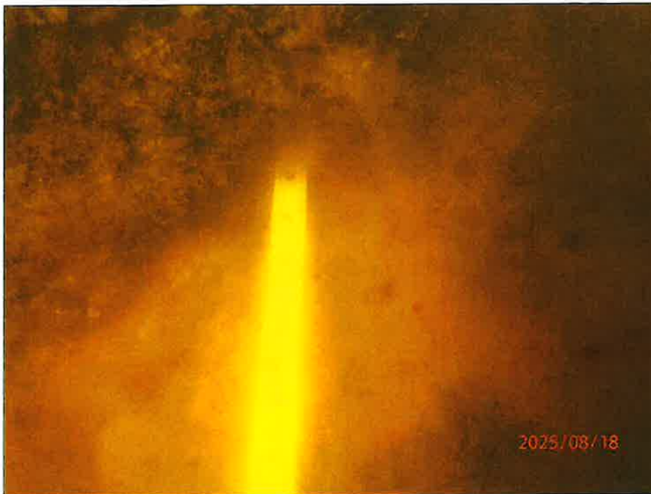
Photo 24 – Void at the northwest seawall, 2 nd , 3 rd and 4 th panels from abutment.
