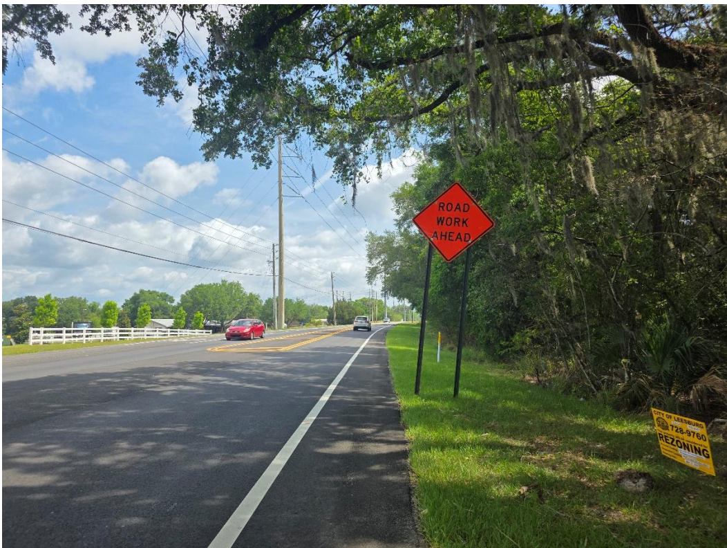
Looking North along County Road 44 from Subject Property.
