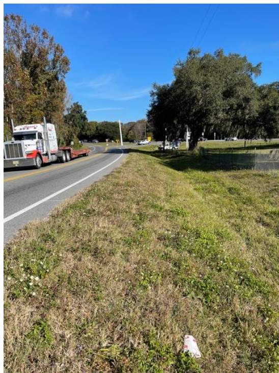
Picture taken from sign posting, looking north along County Road 33 right-of-way.
