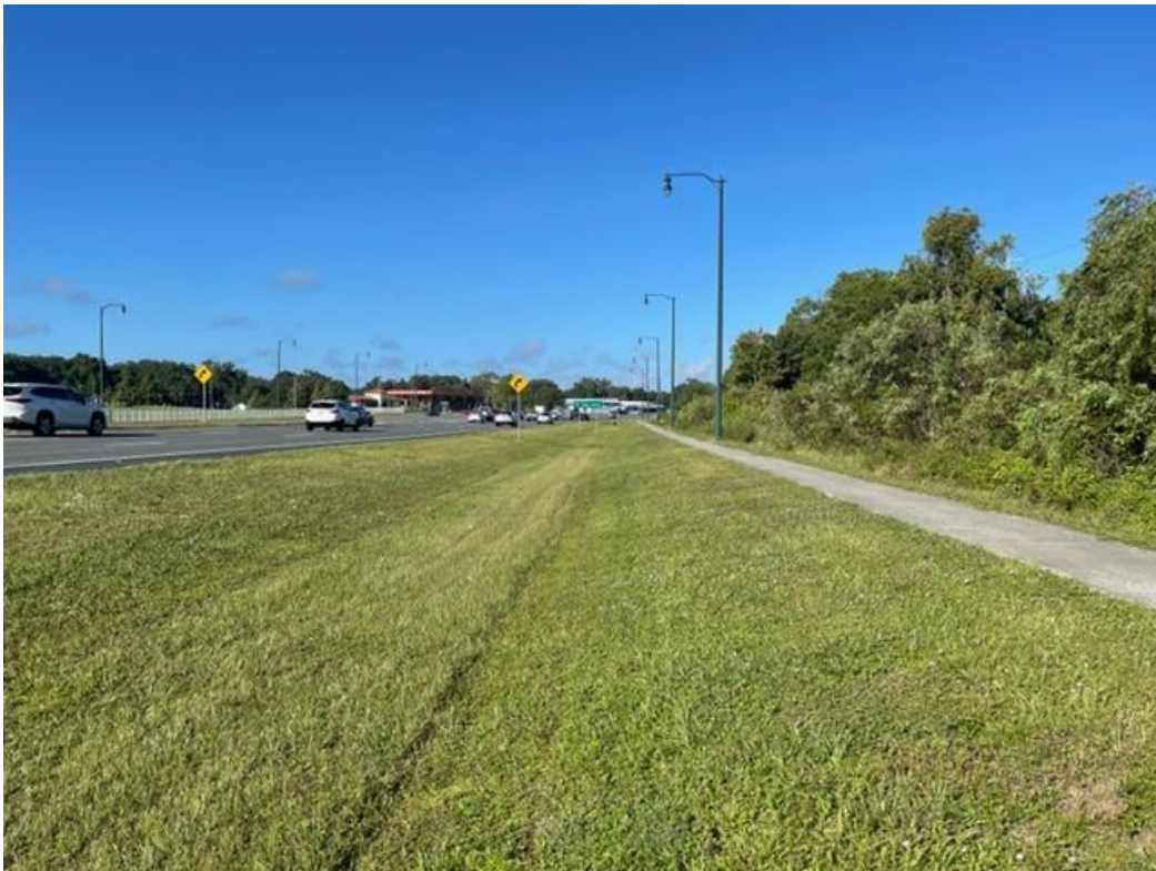
Looking west on US Highway 441
