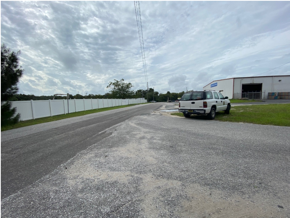
Looking south along North Lake Avenue from sign posting.
