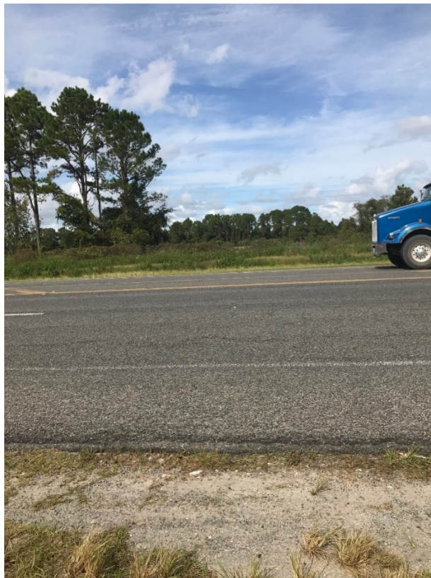
Looking north across C.R. 470 from sign posting.
