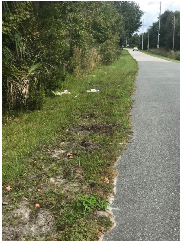
Looking north-easterly along CR 25A from sign posting.
